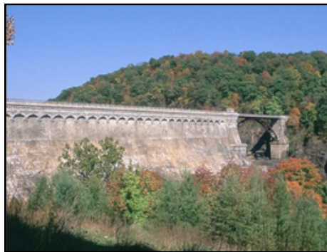
Croton Aqueduct – Photo: aqueduct.org/
