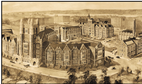
City College Campus - Photo: CUNY
