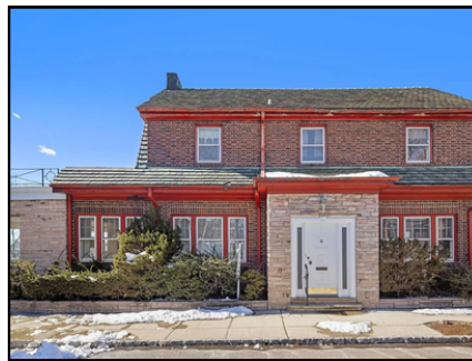
House in Weehawken – Photo: Zillow
