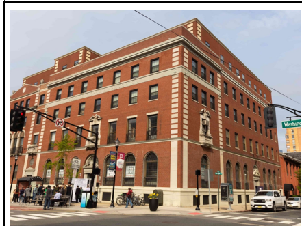
Community Center - Photo: Hoboken Community Center
