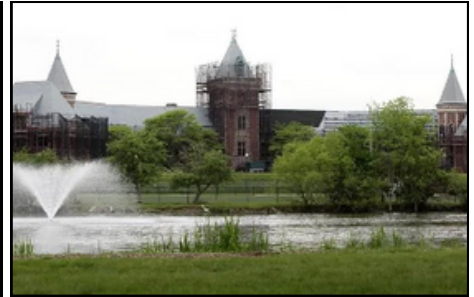
New Rochelle High School - Photo: Google
