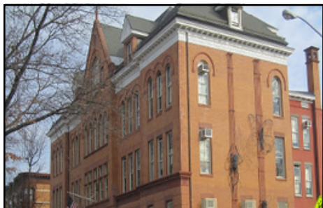
P.S. 107 Public Elementary School - Photo: Google
