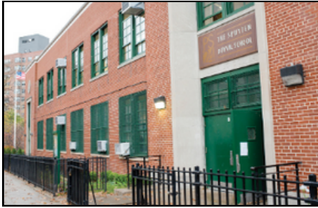
Public K-5 Elementary school – P.S. 24 - Photo: Google
