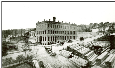
Otis Elevator Factory, 1968 – Photo: Otis Elevator Co., on X (formerly Twitter)
